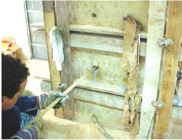
Figure 3: Column confinement with AFRP rods
